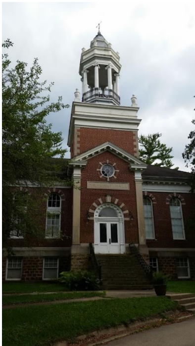
Metcalf Hall. One of the buildings on the IPSC Campus.
